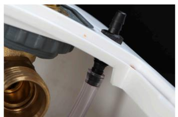
Check that the hose to the connector in the cistern lid and is secure.
